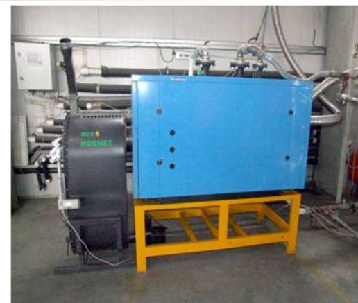
Arzator tip injector ecoHORNET montat pe cazan pe gaze Buderus Eficienta gaze 78%/145kw Eficienta peleti 95%/200kw
